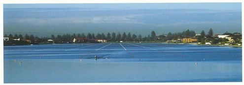
The late 1970s saw the design and construction of a course buoying system that, along pontoons for a held start, and a stretch of water eight lanes wide, 2400m long and at least 3.5m deep enabled the course to gain FISA accreditation. This qualified the course and on shore facilities to be considered for national and international events such as the World Masters Rowing Championships held on the course in 1997.
